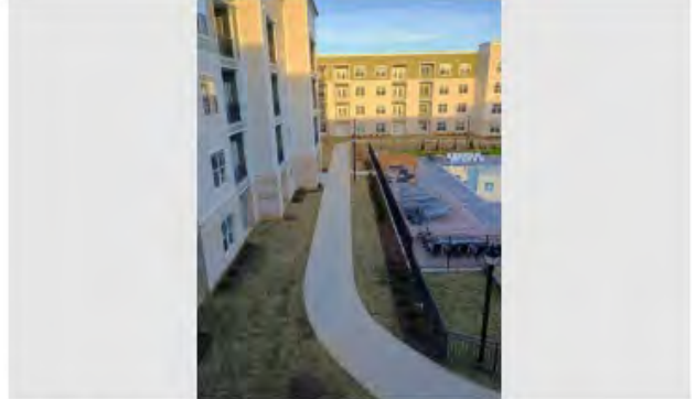
Description Courtyard Sod and Site lighting
