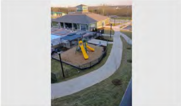
Description Courtyard sod and site lighting
