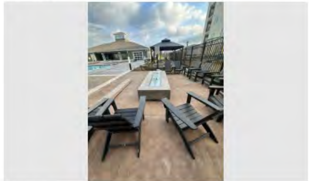
Description Fire Pit Installation
